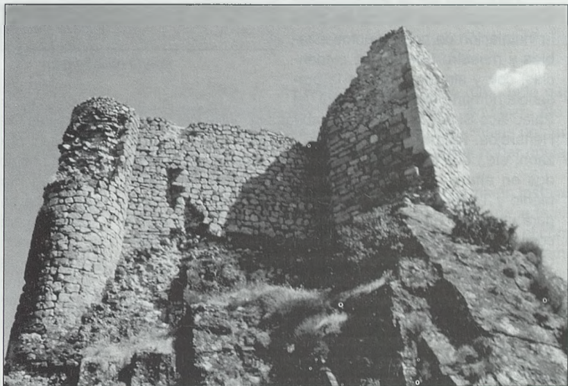
Vista general norte
